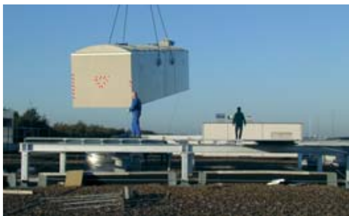
Installation of a bio-filter unit on top of the manufacturing building in Dortmund (Germany)
