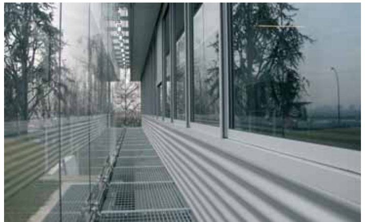
View of double wall and walkway.
